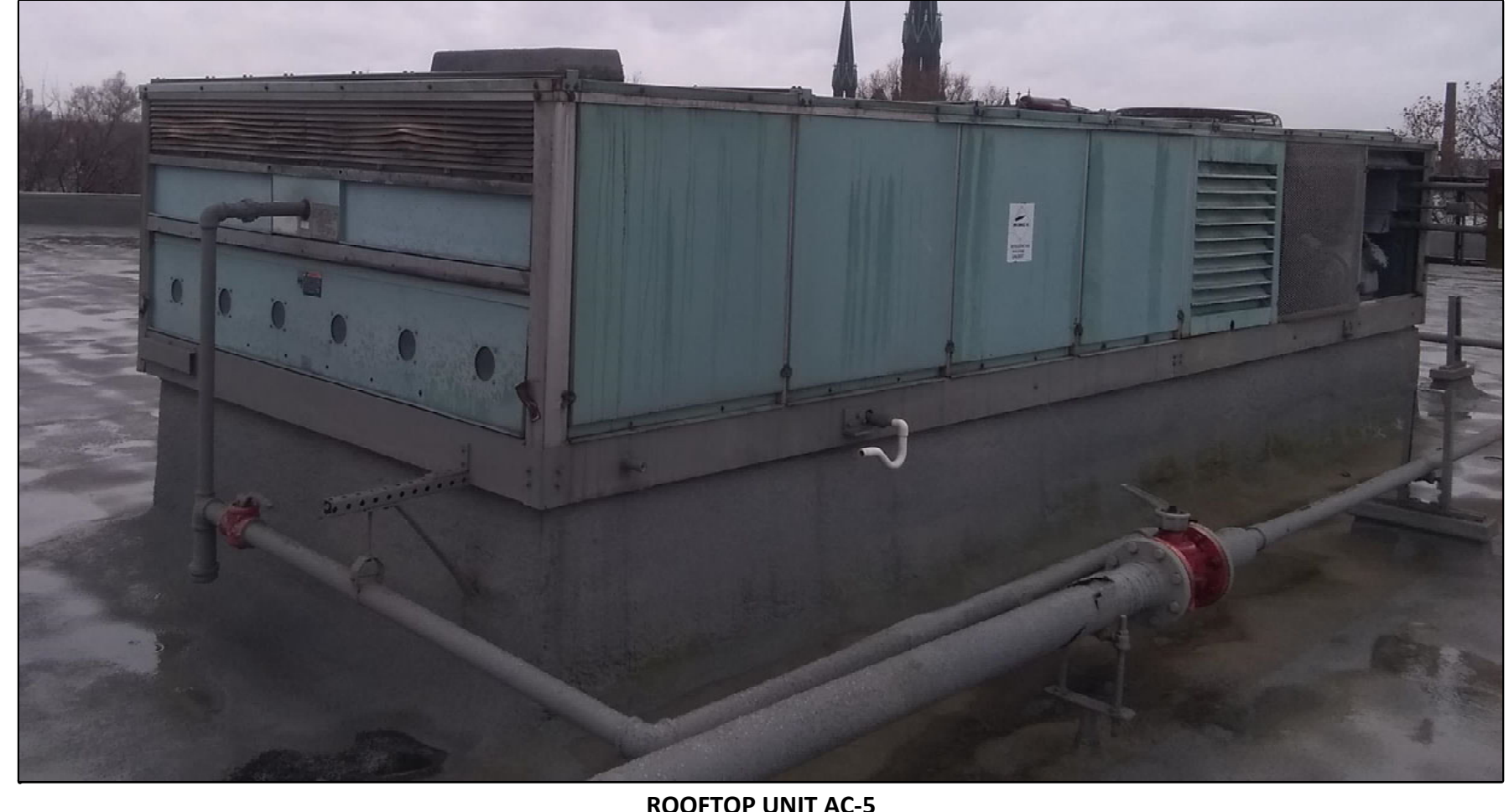
ROOFTOP UNIT AC-5
